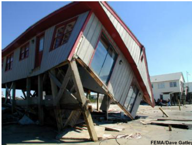
Although elevated, this house in North Carolina could not withstand the 15 ft (4.5 m) of storm surge that came with Hurricane Floyd (1999)
